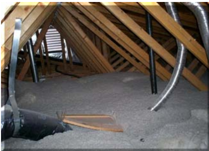
Photo: 9. View of attic. (1)
