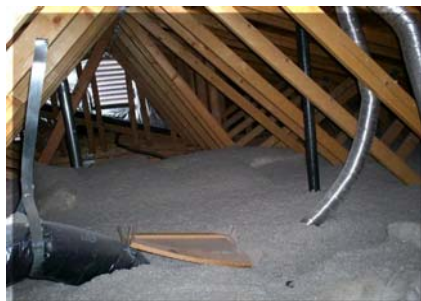
Photo: 9. View of attic. (1)
